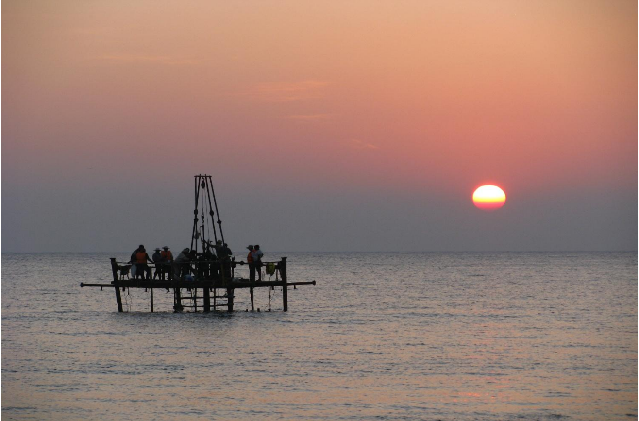
Figure 1: Drilling in Marine
